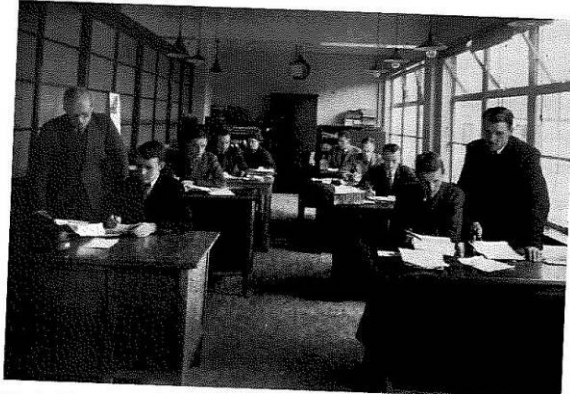
Figure 1, Interior of Building A, circa 1933. Note the steel window on the RHS and internal glazed screen to the LHS.
