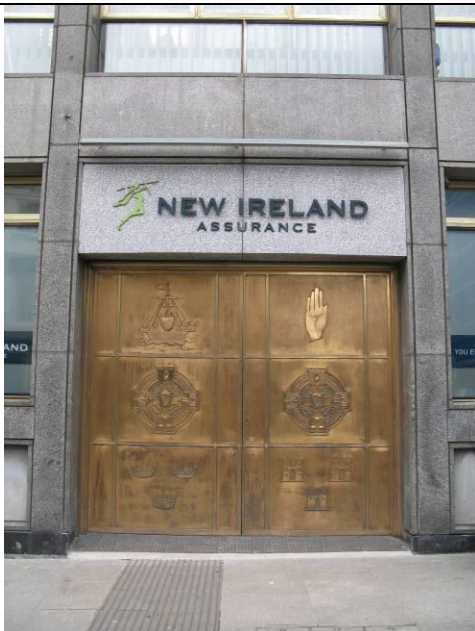
Main entrance door with emblems of four provinces
